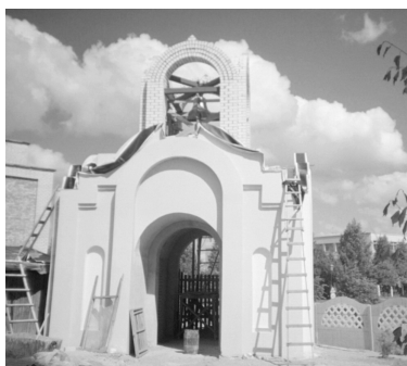
Russian Orthodox Bell Tower being built in Gatava.
